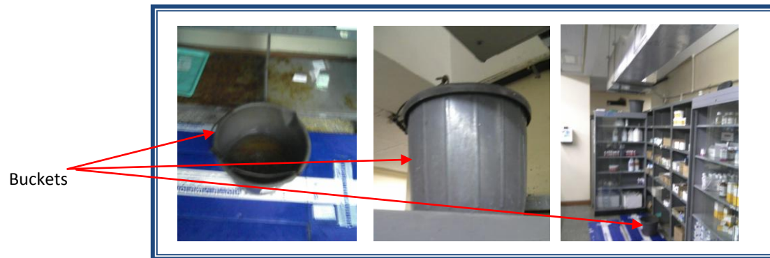
Picture 3 Buckets used to catch water leaking from malfunctioning air conditioning unit at the Cornwall Regional Hospital
