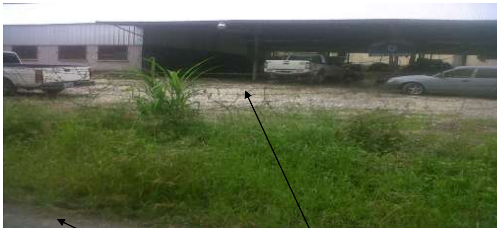
Picture 1 Front View of Area Two Garage, Richmond
